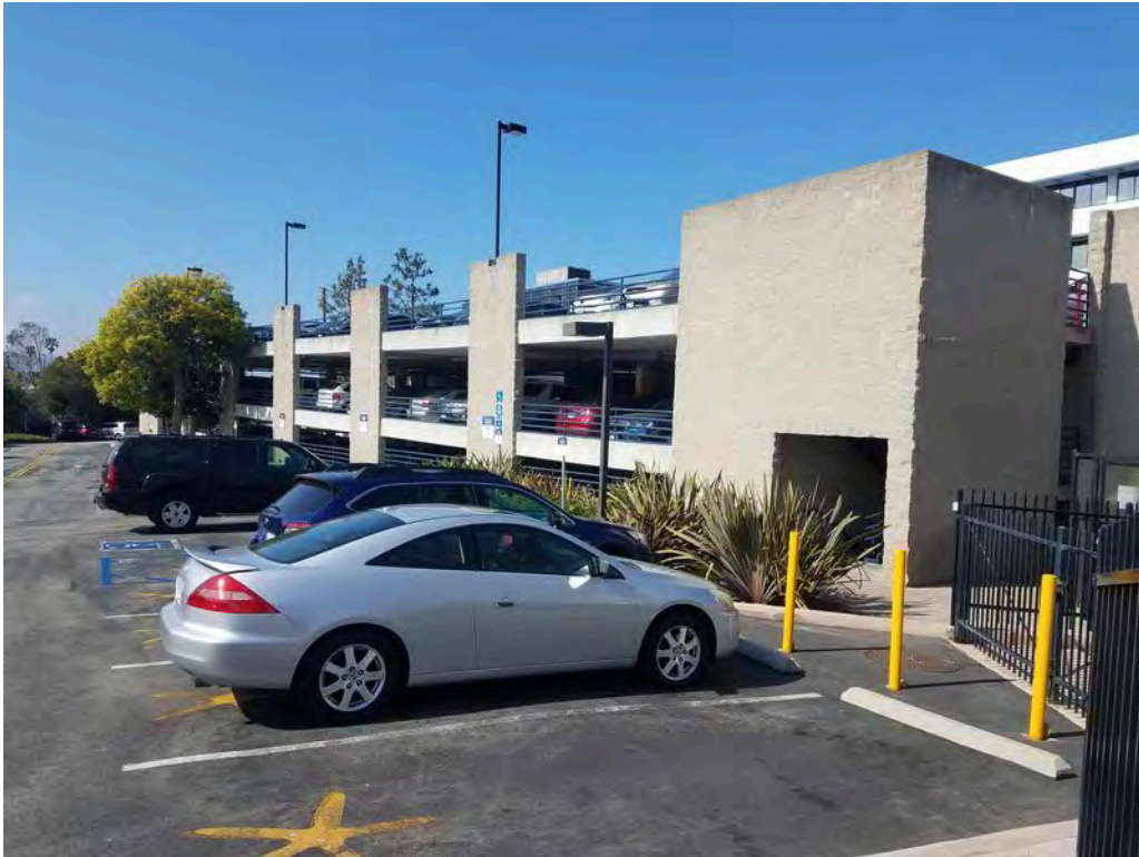
View of above-ground, four-level parking structure.
